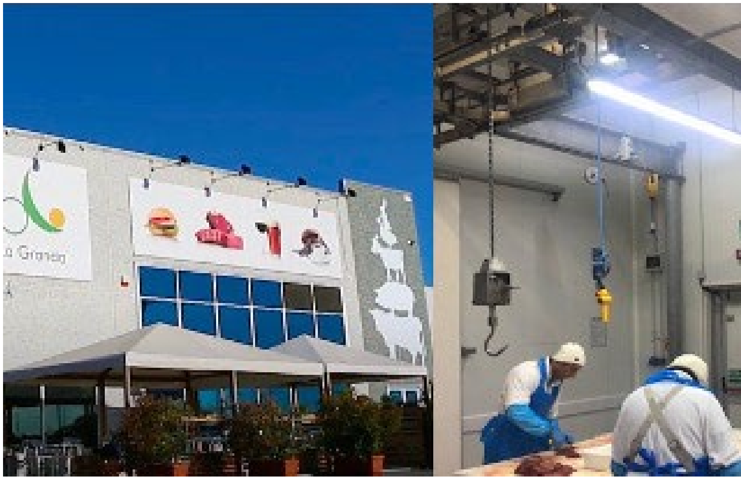
La Granda Plant – Genola, Italy
